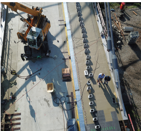
integration drainage into footpath
