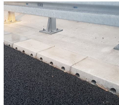
Bridge drainage units from the road surface
