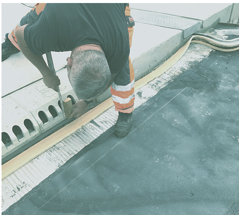
Explanation on site
