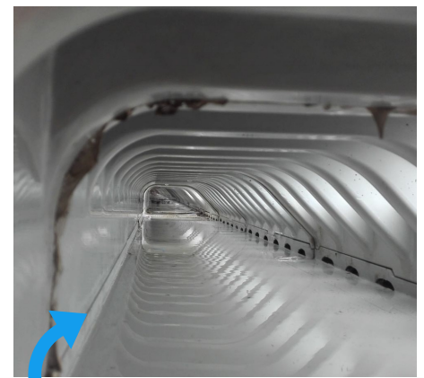
Cleaned Bridge Drainage Unit
