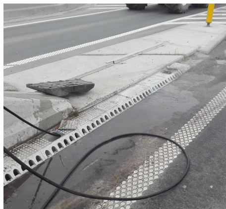
Maintenance by Franki Construct
