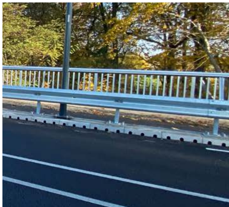
Bridge Drainage on location
