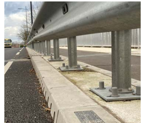
From the roadbed
