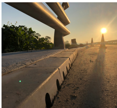
Integratie afwatering in rws detail
