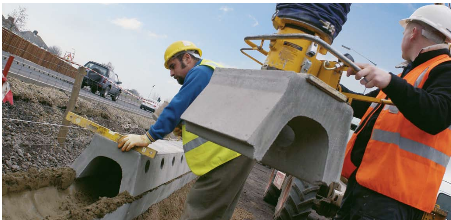
Beany Block installation, mechanically handled
