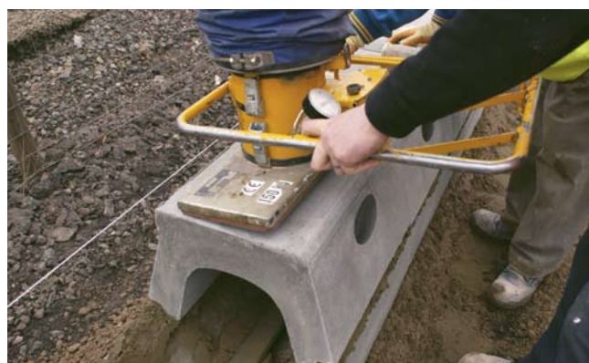
Beany Block installation, mechanically handled
